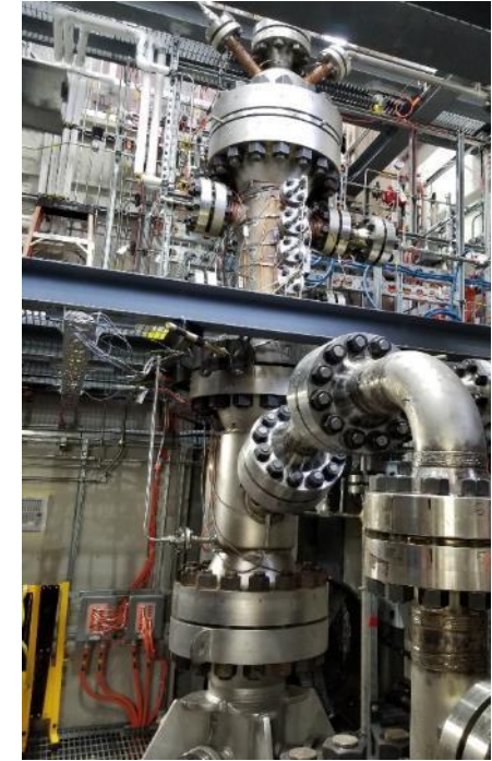
Three-storey high oxy-combustion pilot plant designed to operate at max 85 times atmospheric pressure for steam/heat/power generation with high efficiency and near zero emission
